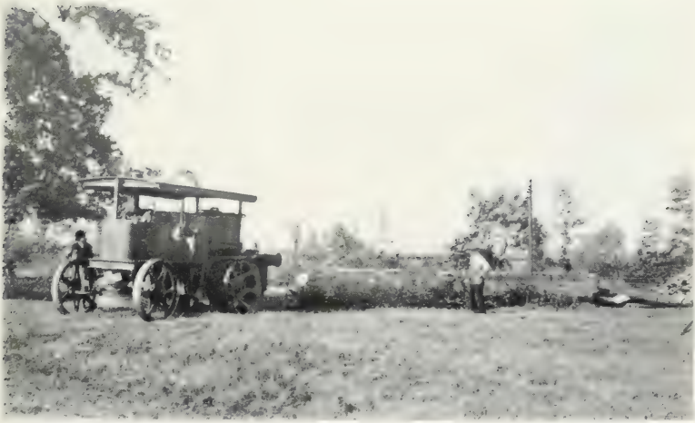
FIG. 44. STEAM WAGGON'S WINCH DRAGGING LOG OUT OF HOLLOW.
